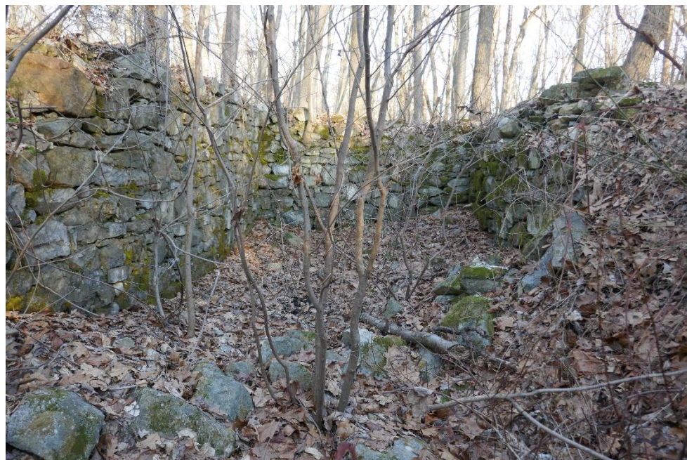
Figure 14. The right wall of this feature is the end of the tramway roadbed.
