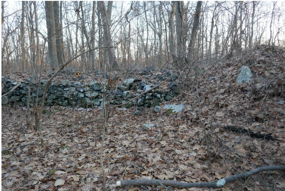
Figure 13. Tramway roadbed adjacent to the roadbed end point.
