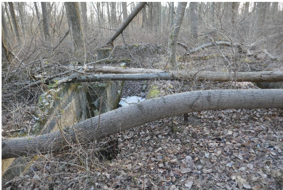
Figure 2. Concrete foundations at 1939-1943 magnetic ore concentrating plant.
