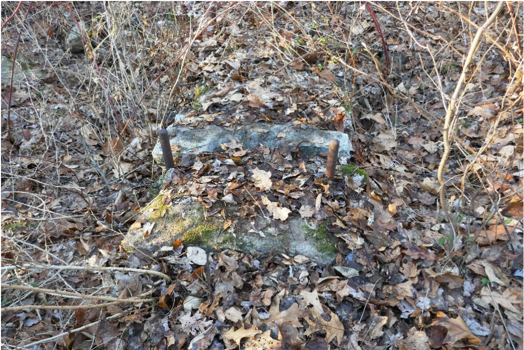
Figure 19. Threaded bolts set in stone.
