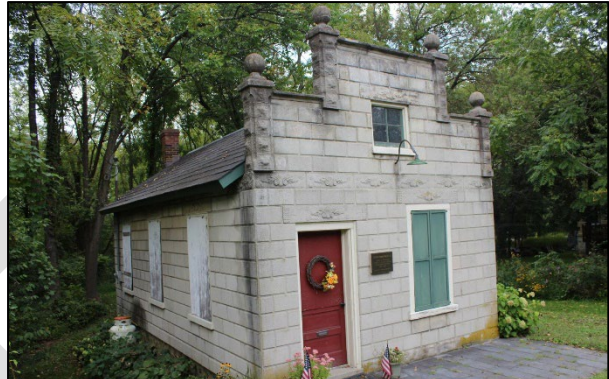
Figure 2 - West Portal Old Town Hall, located along Brunswick Pike.
